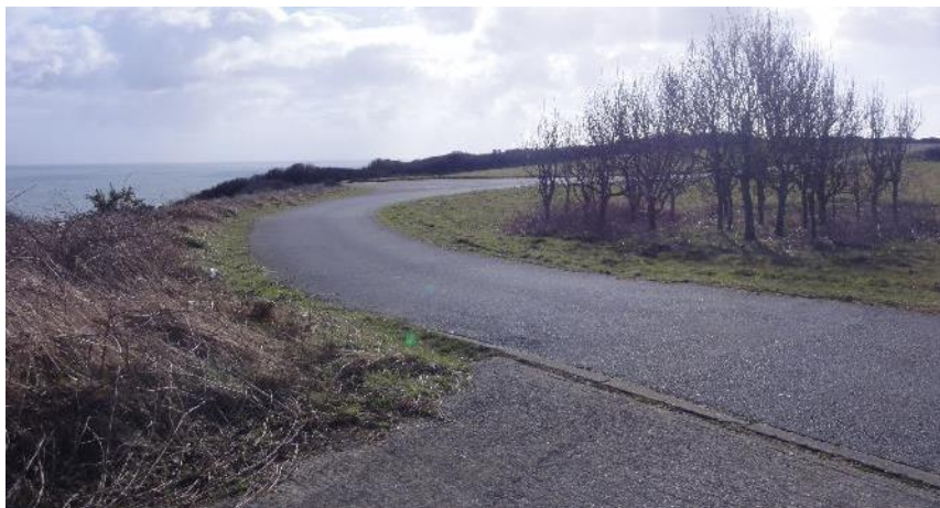
Figure 5.6 - Approaching the viewing area
