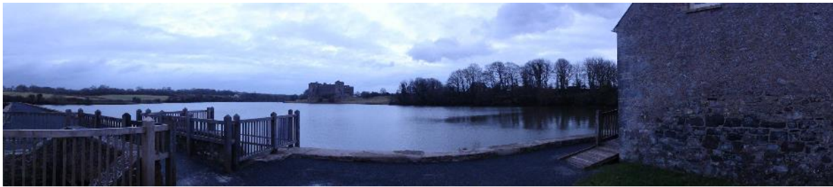
Figure 5.35 – View east towards Castle
